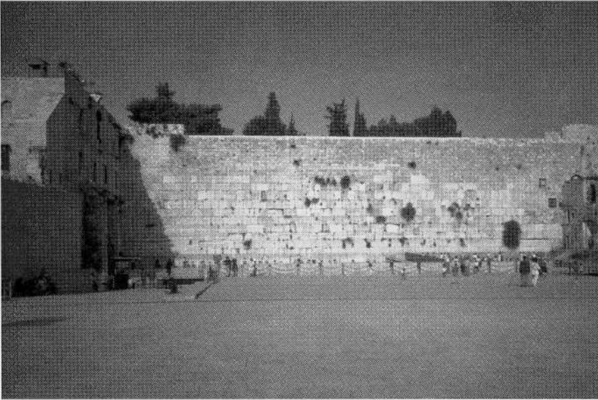
Illustration 1.3 The western retaining wall of the Herodian temple—known as the Wailing Wall.
